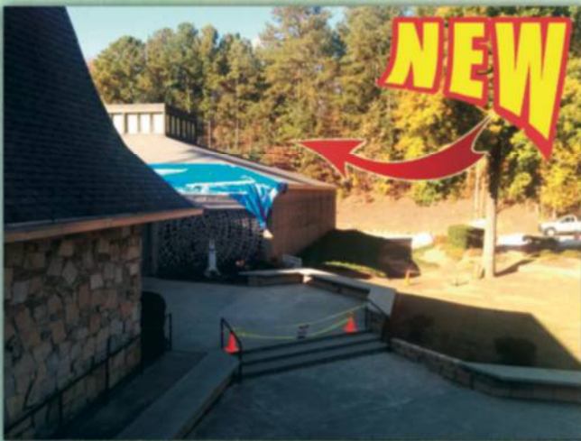
Photo on the left: New roof has been installed on the east side of the church!
